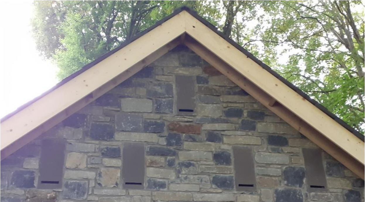
Plate 4: Close up of Bat Tubes inserted in external walls of bat house constructed in 2021.
