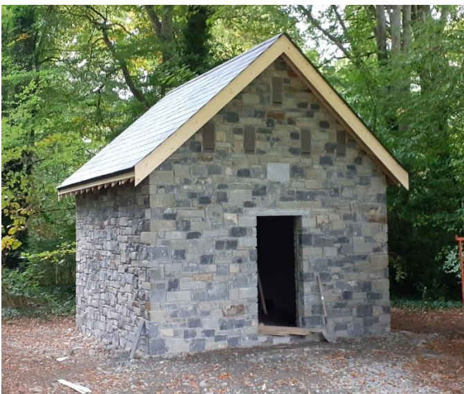
Plate 3: Example of bat house constructed in 2021 (Internal space 4mx4m).
